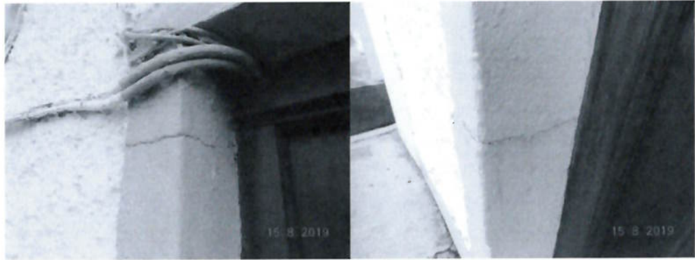
Slight cracking to reveals of front main entrance door.
