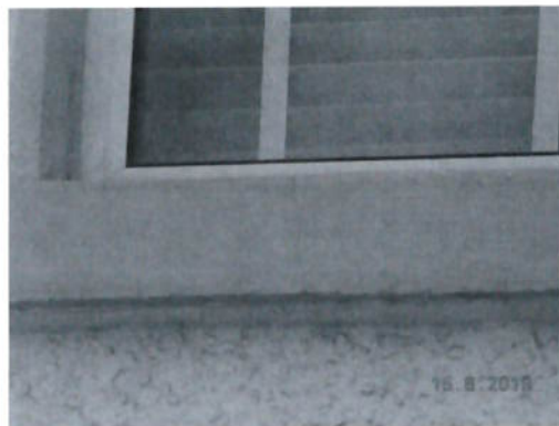
Very fine cracking through the first floor level window cills as viewed from the front elevation.
